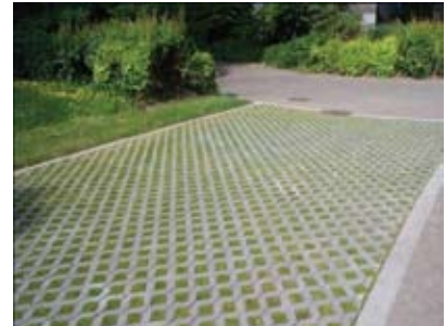
Fig 3: Paves surfaces with grass
